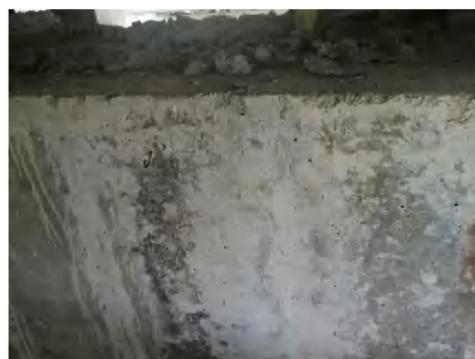
桥墩盖梁竖向裂缝
